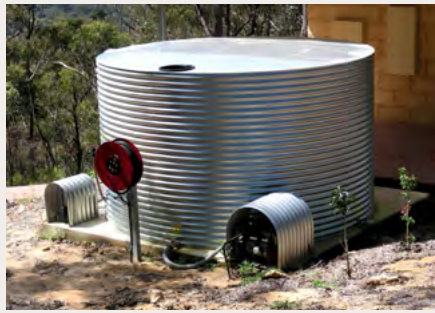
↑ Active fire defences can include metal or concrete water tanks with a diesel pump and a hose long enough to reach around the property.
